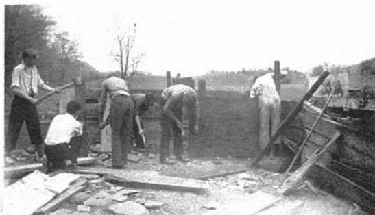
LEFT - AG. BOYS WORKING ON HOWARD TURNBULL'S HOG HOUSE.
