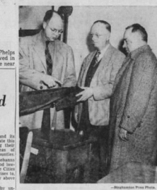
DEADLY FIRE—Assistant Fire Chief Arnold Rollins, left, points to holes in smoke pipes recovered from ruins of a rural residence near Edinburg where three persons were killed. Coroner Joseph Phelps, center, and Chief Tom Lockrie look on. He said accumulation of cinders in pipes caused fire which claimed three lives yesterday.
