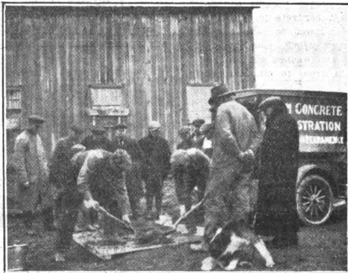
Cement Demonstration at Farm of Henry Williams, Bennettsville, N. Y. These Demonstrations were Available for Every School District through The District Committeeman.
