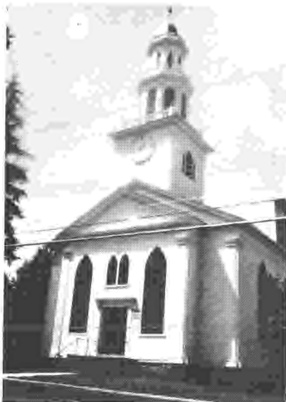
The Presbyterian Church built in 1833 by the Rockwell brothers, later a Village Hall, a Town Hall, and since 1958 the Grange Hall.
