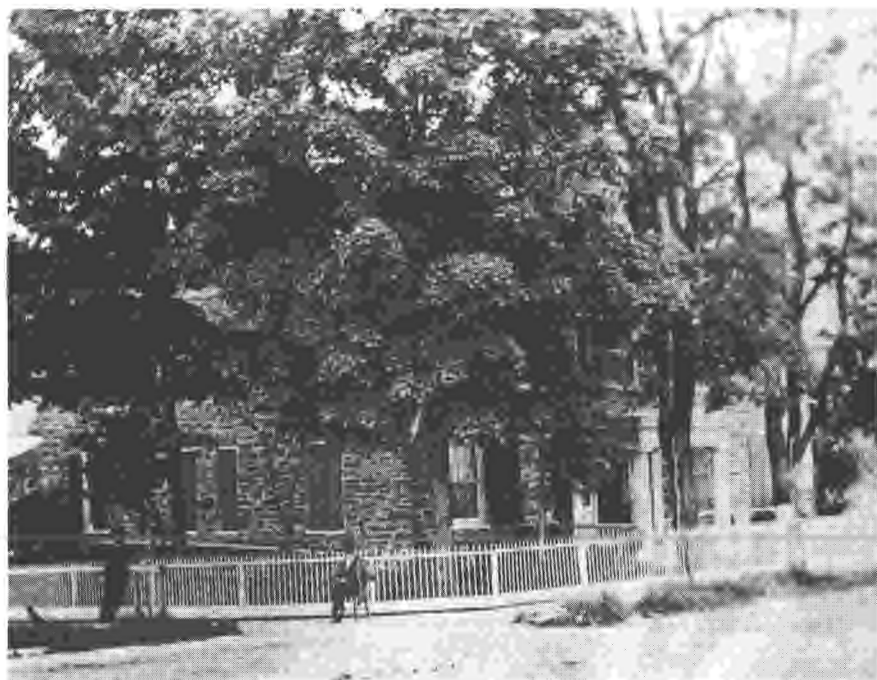
The Gilbert Homestead, built by Joseph T. Gilbert in 1822 and destroyed by fire in 1895.
