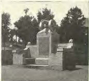
MONUMENT PARK, RICHFIELD
