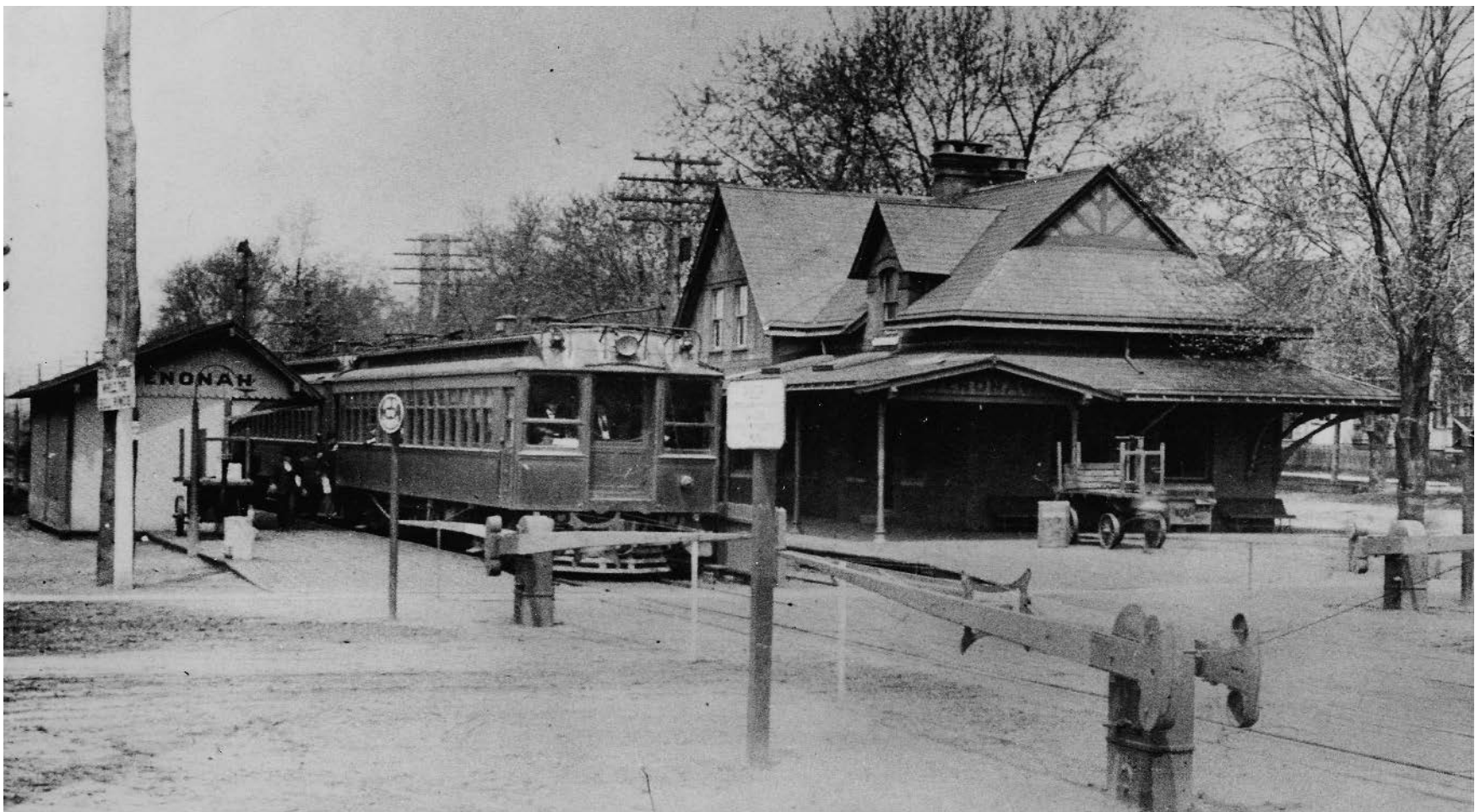
Train Station - Current Location on East Side of Tracks
